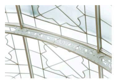
For safety reasons (a piece of broken glass falling down 18 metres is a fatal weapon!), the windows were given double glazing during the restoration work. First, a negative of each pane was made. Then, the original panes and the replicas were joined together by a layer of resin so as to produce the double glazing.
